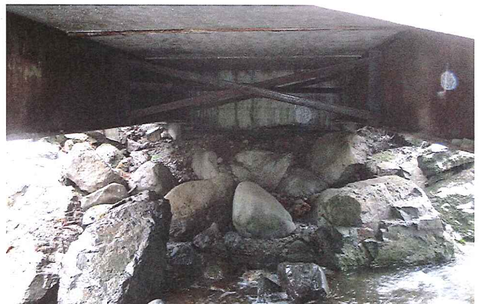
CK-2040 Abutment Right Bank
