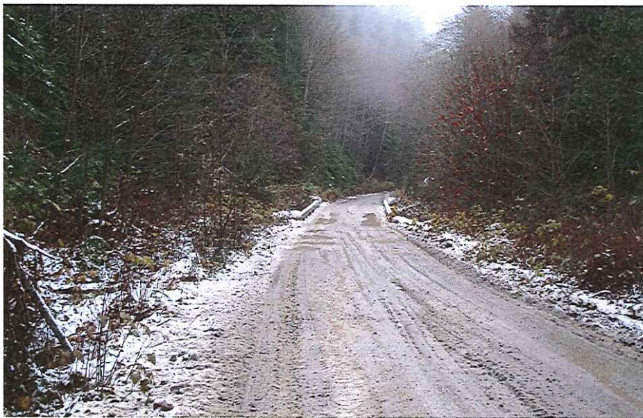
CK-2040 Approach Right Bank
