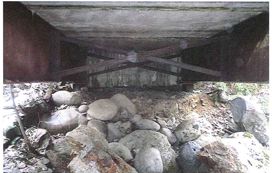
CK-2040 Abutment Left Bank
